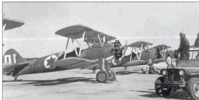
Above Left: Boeing PT-17 Stearman no.2701 is seen in 1949-1950 brown and green over Light Mediterranean Blue scheme, with RAL1032 (FS33637) Trainer Yellow identification stripes applied to the fuselage and wings. The Stearman served as the IAF's primary trainer for 15 years until its replacement by the Piper model PA-11-95 in 1960. The Stearman had a four-digit number applied starting with the number 27. The last two digits of the number were applied to the top of the right wing, bottom of left wing, and to both sides of the rudder, with the full four-digit number applied to the sides of the fuselage.
